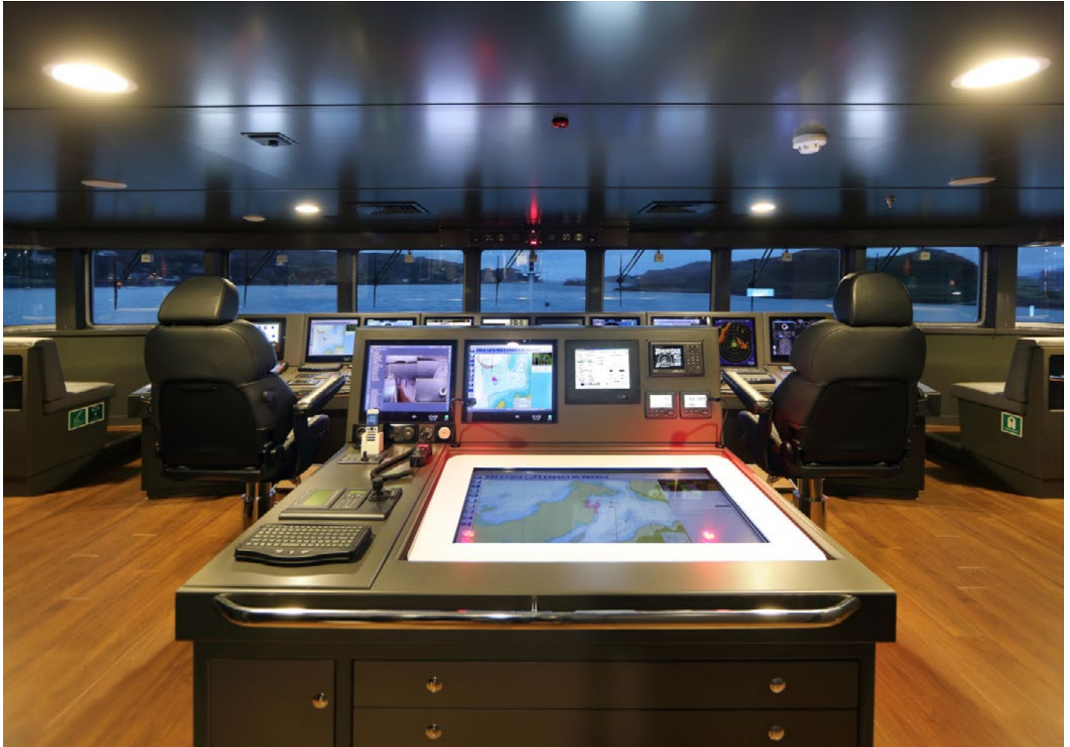
BRIDGE DECK - ECDIS NAVIGATION CONSOLE
